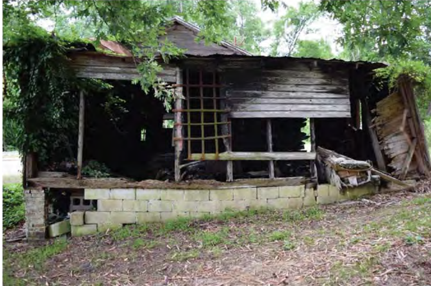
Figure 13: Willie F. Parker Service Station, west (rear) elevation, facing east
