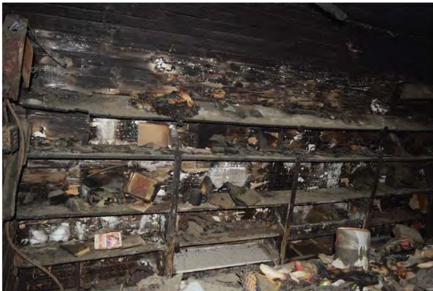
Figure 14: Willie F. Parker Service Station, south interior wall, facing south
