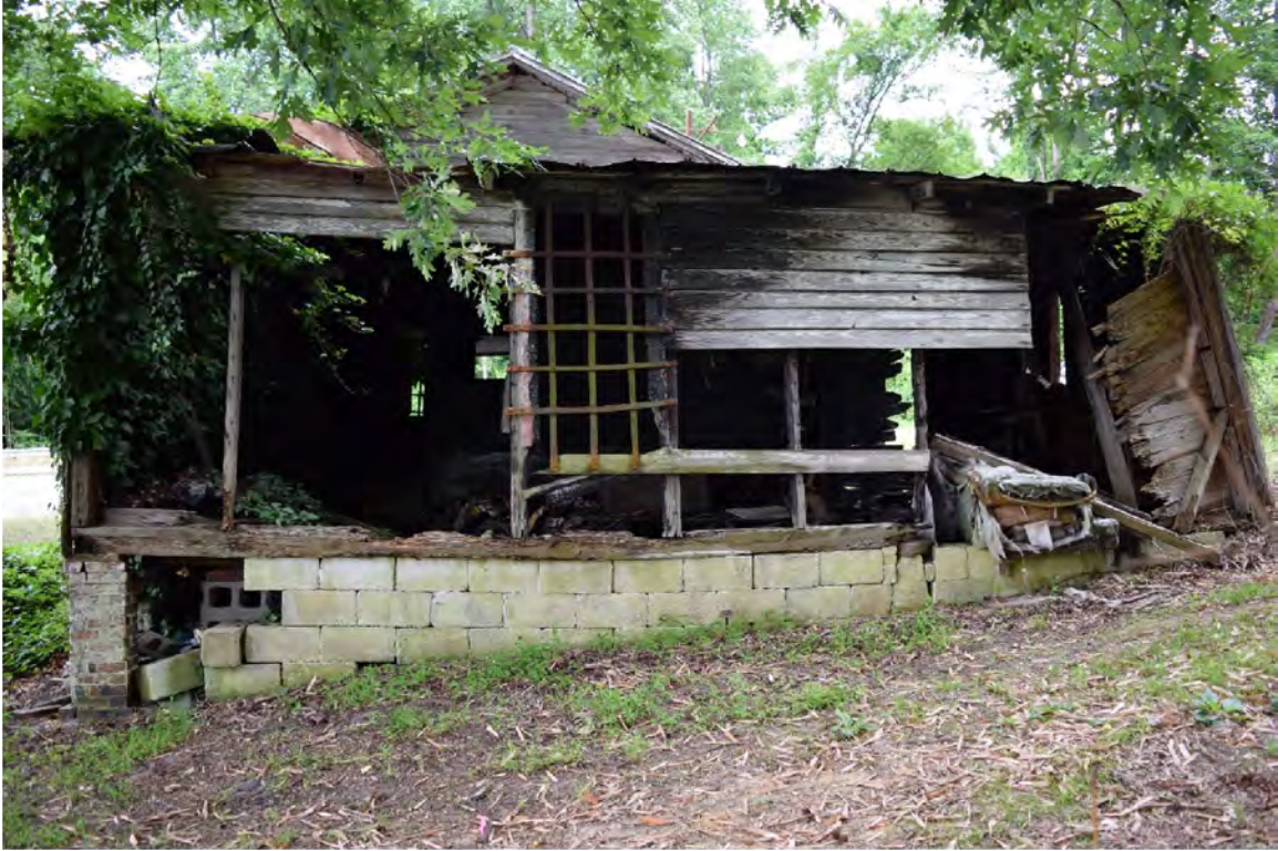
Figure 8. Willie Parker County Store, addition 1 (left) and addition 2 (right), west elevation.
