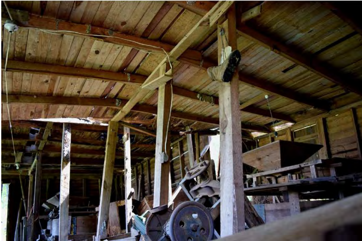
Figure 26. Millhouse addition ceiling view from the double-door entry.
