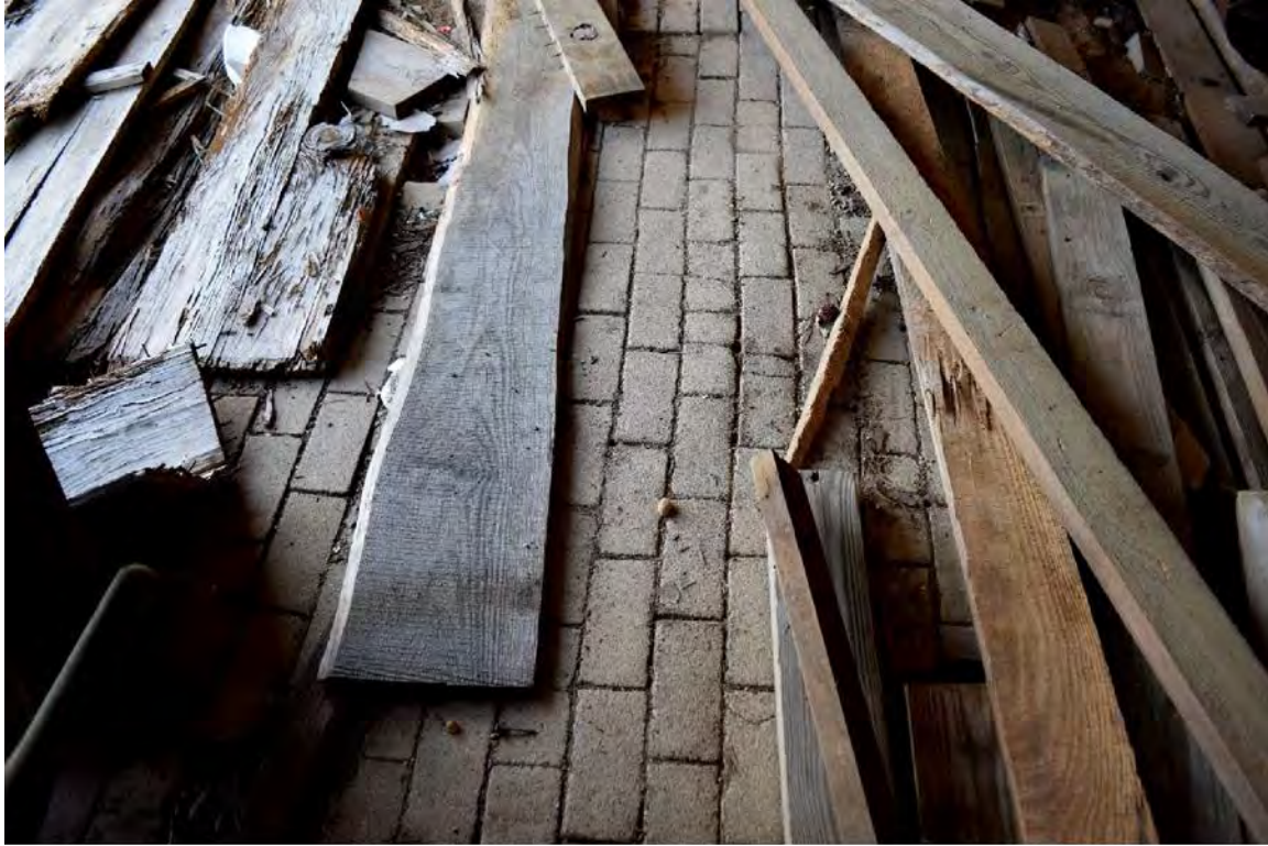
Figure 20. Millhouse addition, concrete paving brick floor detail.
