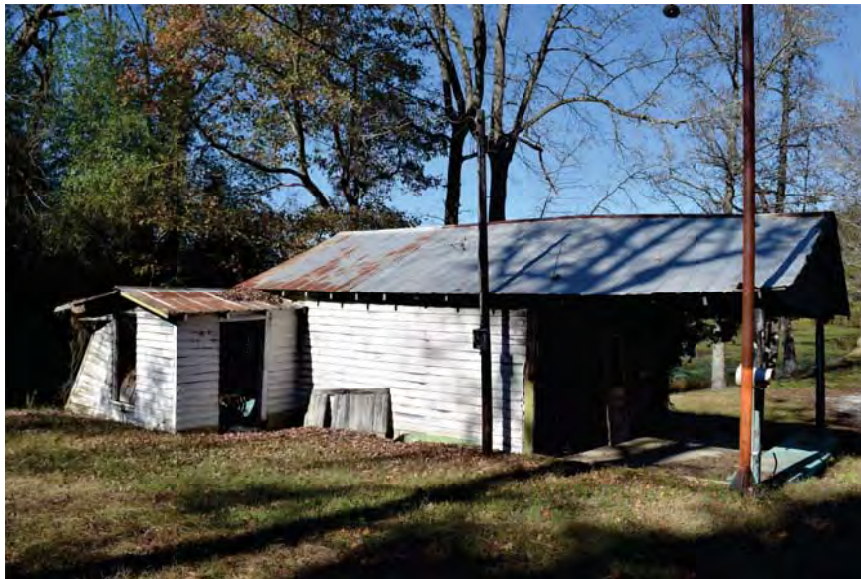
Figure 12: Willie F. Parker Service Station, facing northwest
