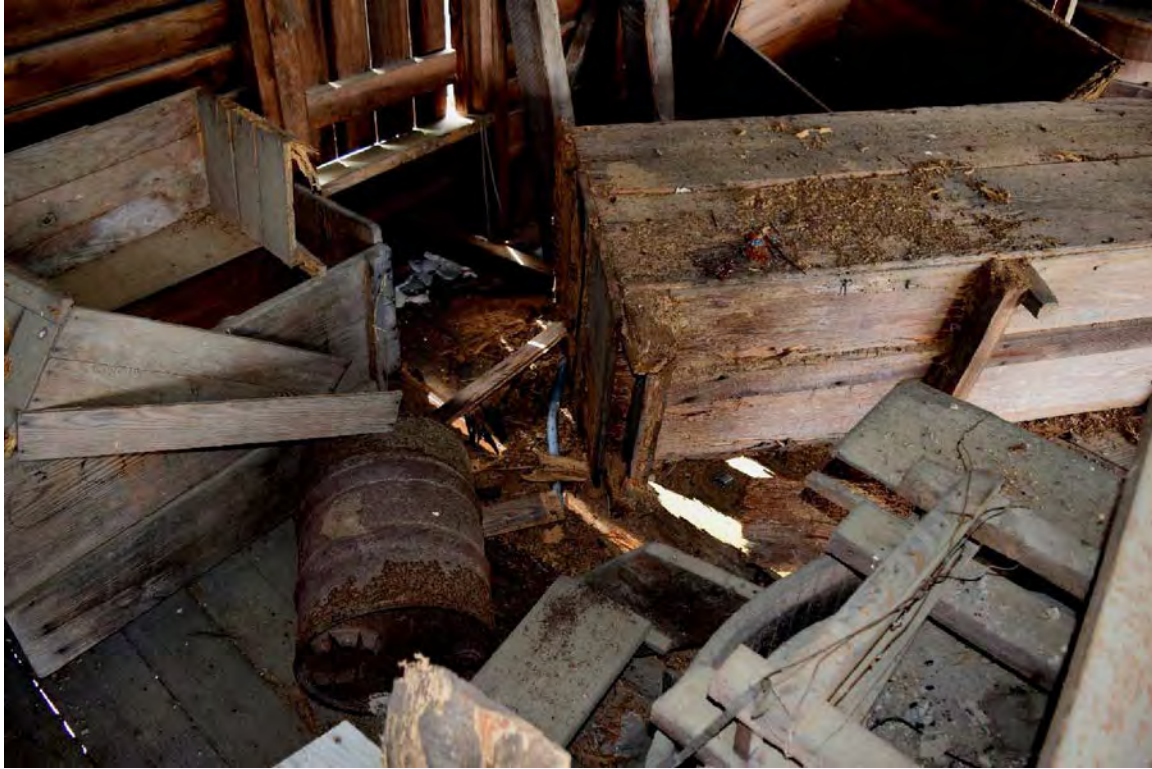
Figure 34. Original millhouse interior, northeast corner showing cornmeal bins along the east wall and near one of the wooden-shuttered windows of the original mill house.
