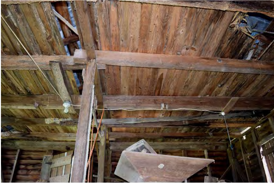
Figure 35. Original millhouse interior, ceiling detail, view toward the north wall.
