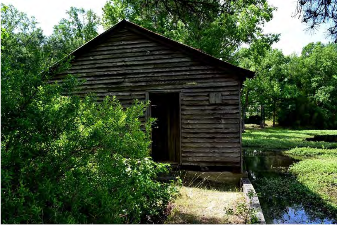
Figure 6. Original millhouse north elevation; Parker Mill Pond on the right.
