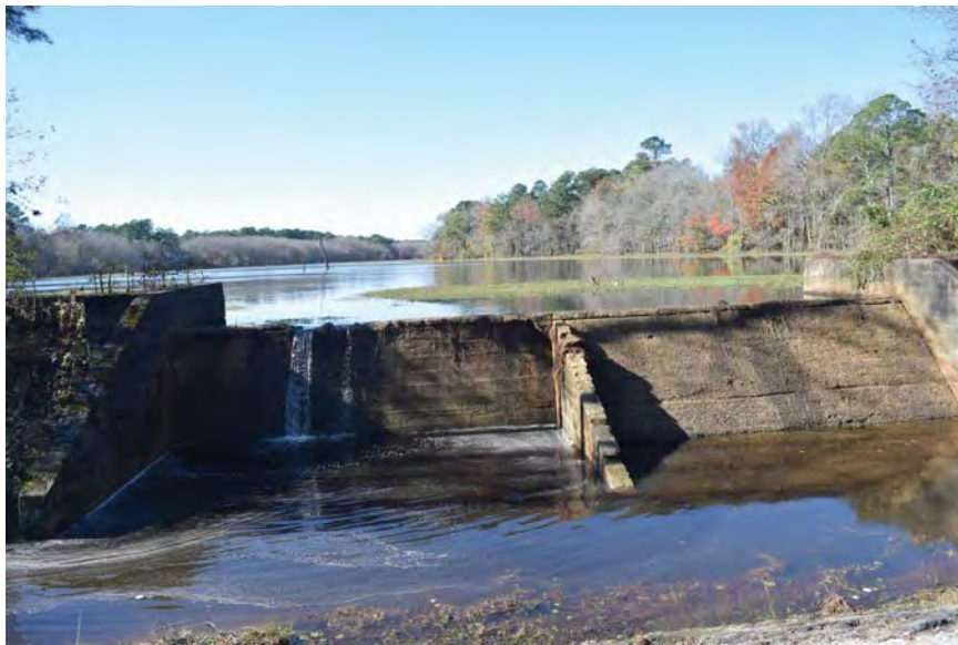
Figure 9: North spillway, facing west
