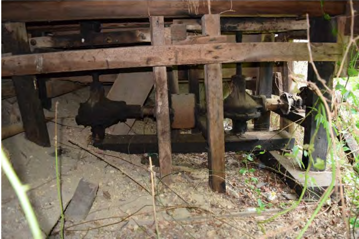
Figure 38. Millhouse addition, Case motor under the building.
