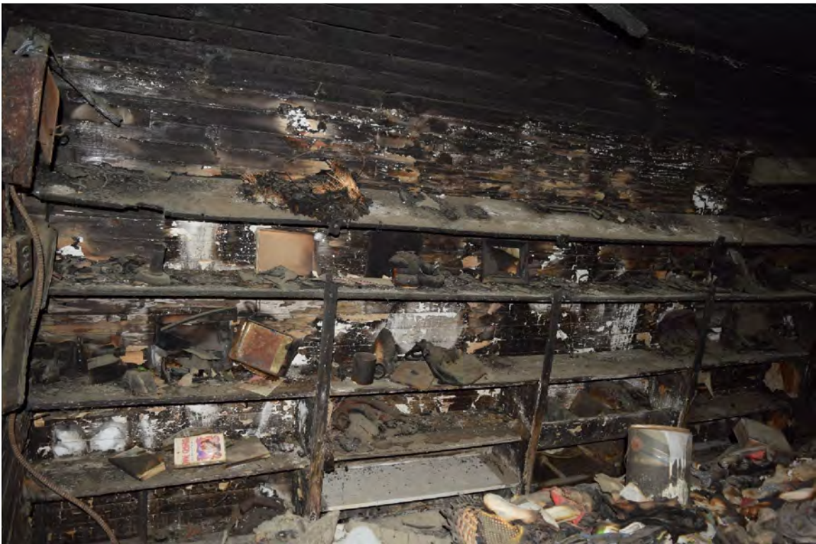
Figure 13. Willie Parker County Store, main structure interior, south wall.
