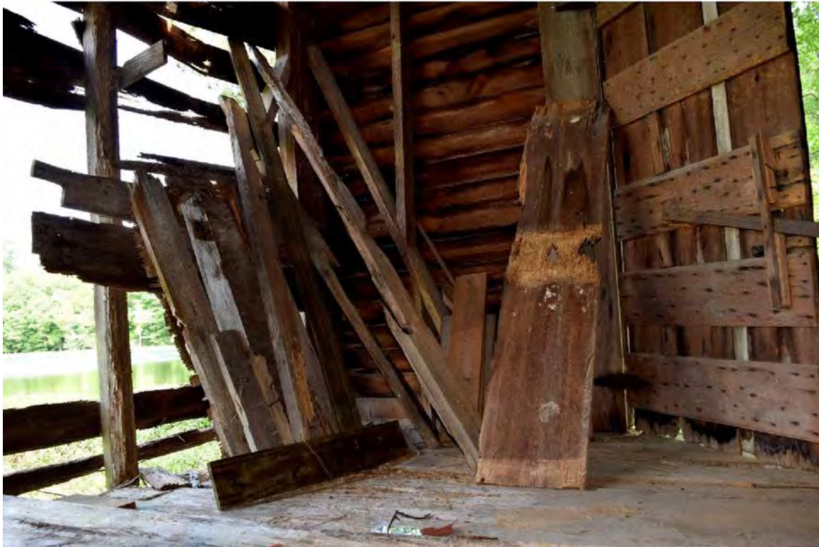
Figure 29. Original millhouse interior, northwest corner showing the batten door.
