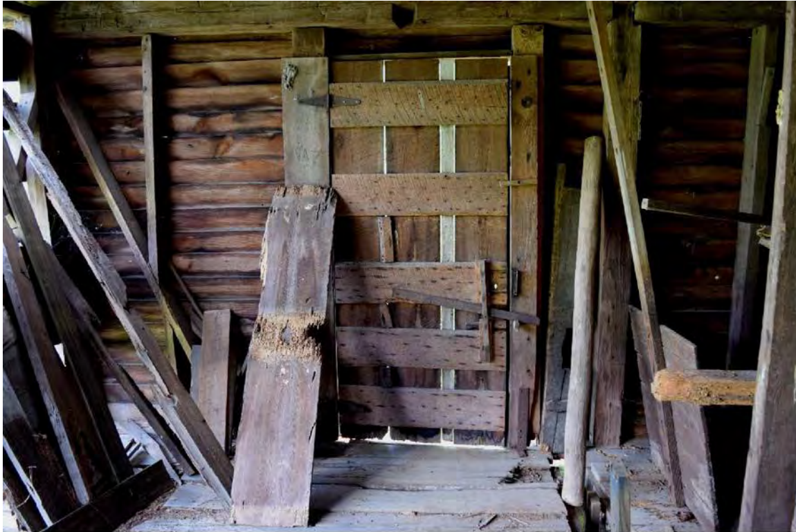
Figure 30. Original millhouse interior, north wall and door.
