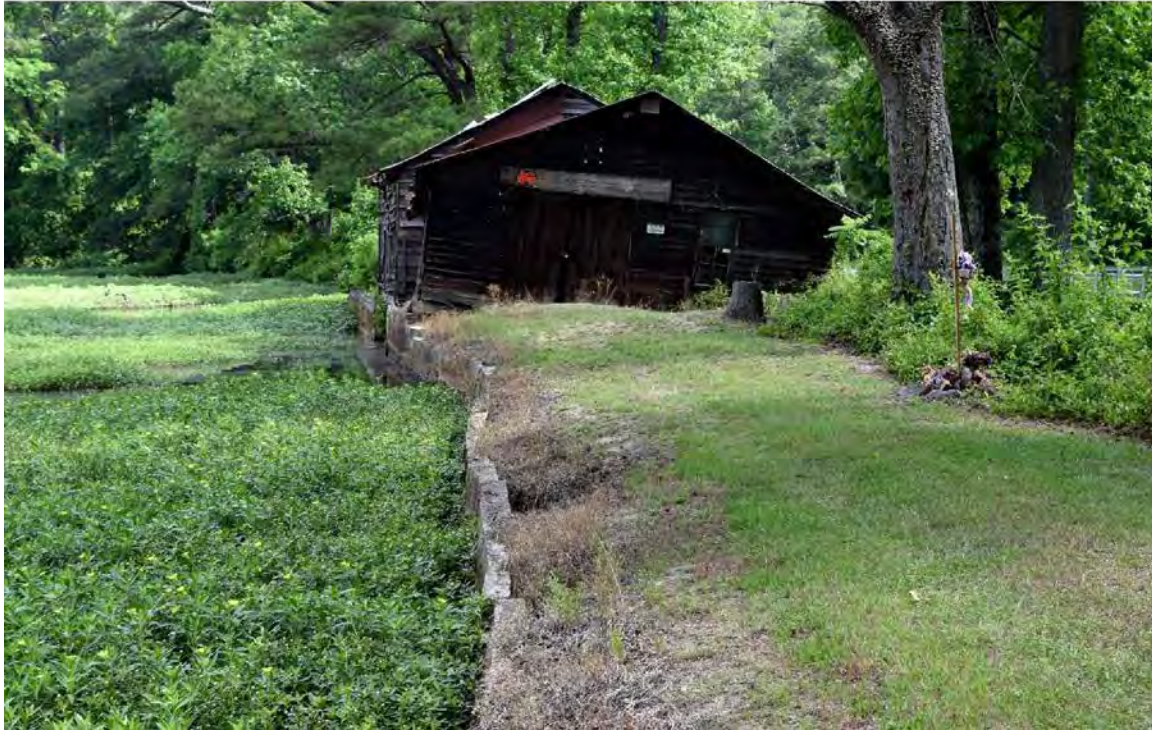
Figure 11. Millhouse addition south elevation showing the concrete retaining wall along the earthen dam that was used as a millhouse road; Parker Mill Pond on the left.
