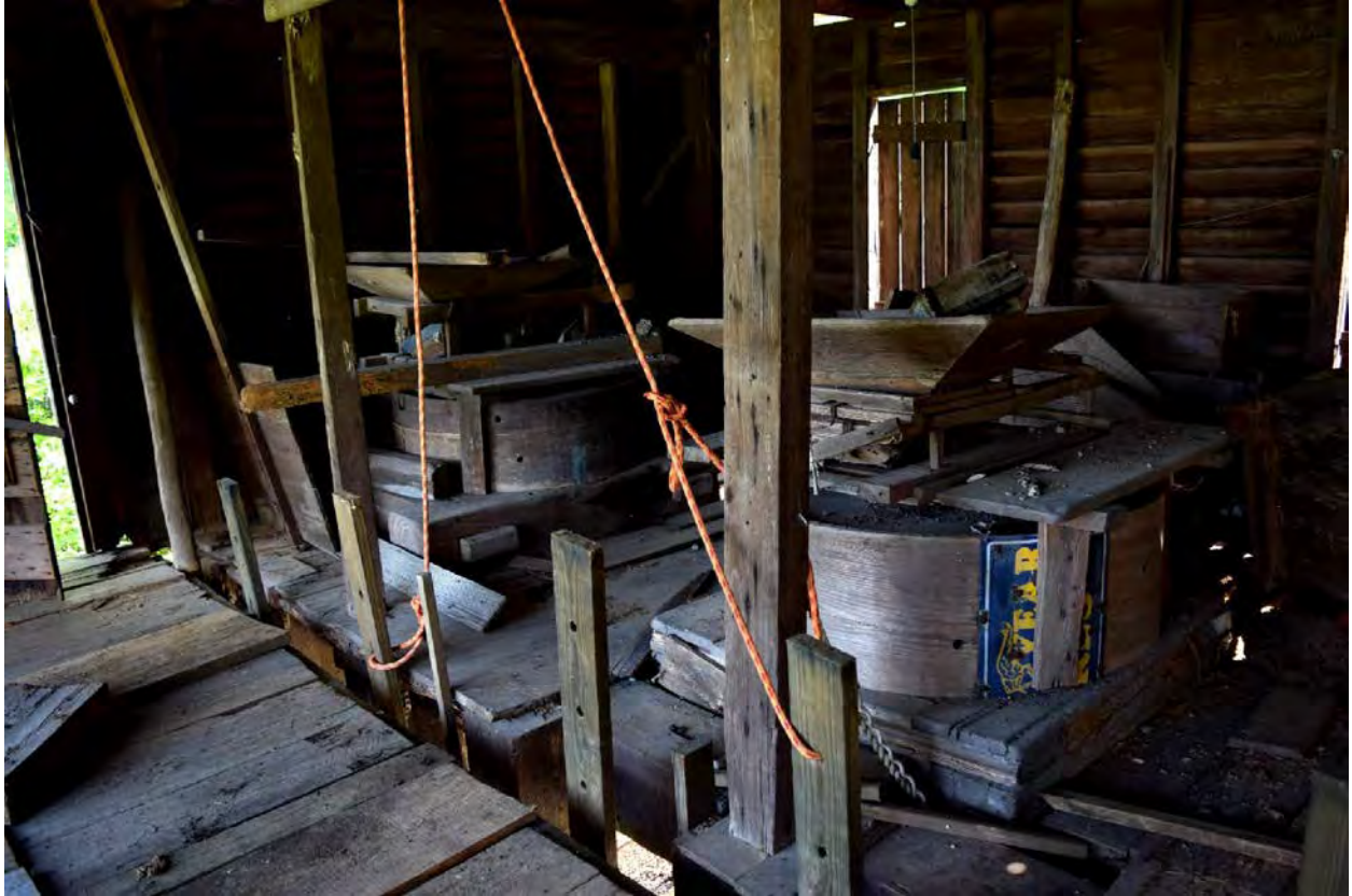
Figure 32. Original millhouse interior, northeast corner showing two corn grinding machines, one of the wooden-shuttered windows on the east wall of the original mill house, and the sluice gate controls.
