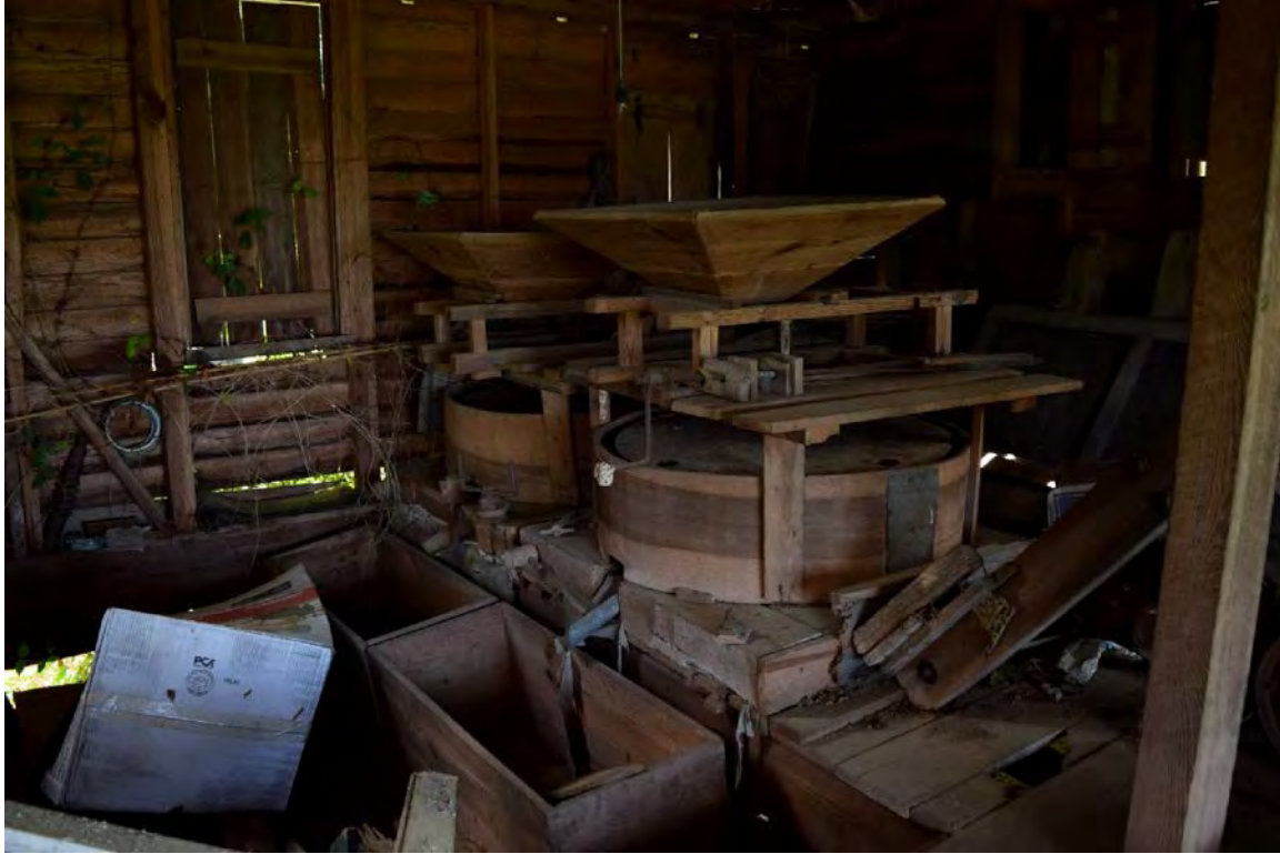
Figure 24. Millhouse addition southeast corner showing the two corn grinders on the entrance level wood floor, the two cornmeal bins on the lower level, and the wooden-shuttered window on the east wall.
