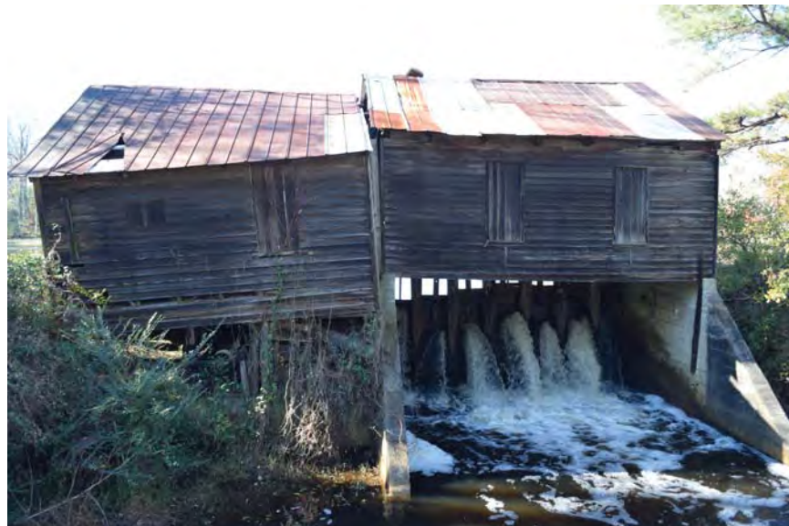
Figure 3: Parker's Mill, east elevation, facing west
