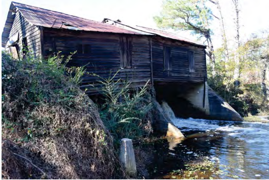
Figure 8: Parker's mill house and south spillway, facing west-northwest
