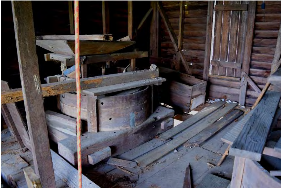
Figure 31. Original millhouse interior, northeast corner showing one of the corn grinding machines and one of the wooden-shuttered windows on the east wall of the original mill house.
