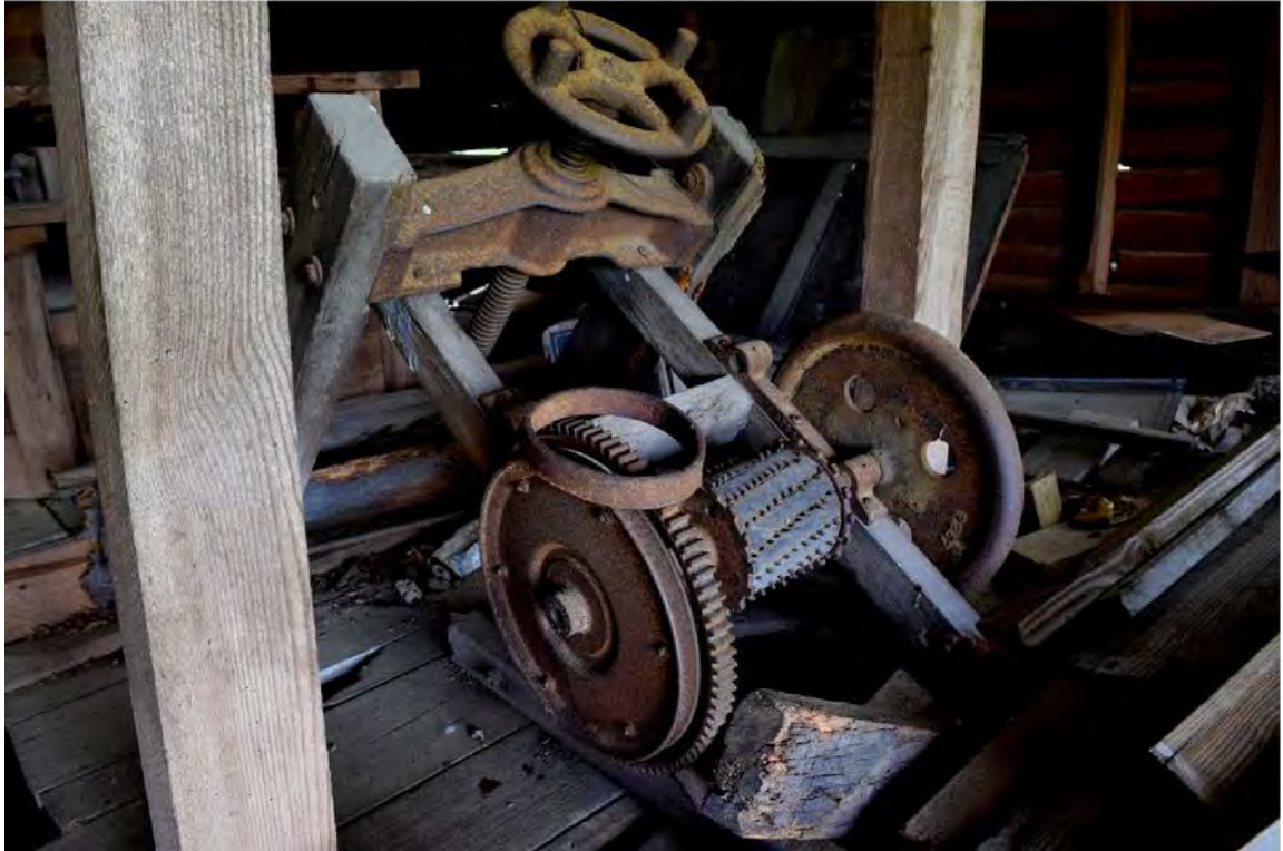
Figure 21. Millhouse addition, machinery on the entrance level wood floor.
