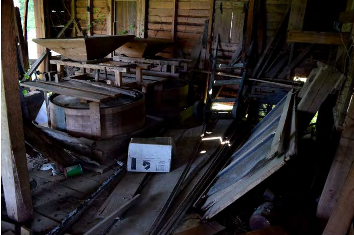
Figure 22. Millhouse addition, view from the double-door entrance toward the northeast corner showing the two corn grinders on the entrance level wood floor.
