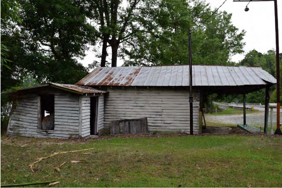
Figure 10. Willie Parker County Store, main structure (right) and addition 2 (left) south elevation.
